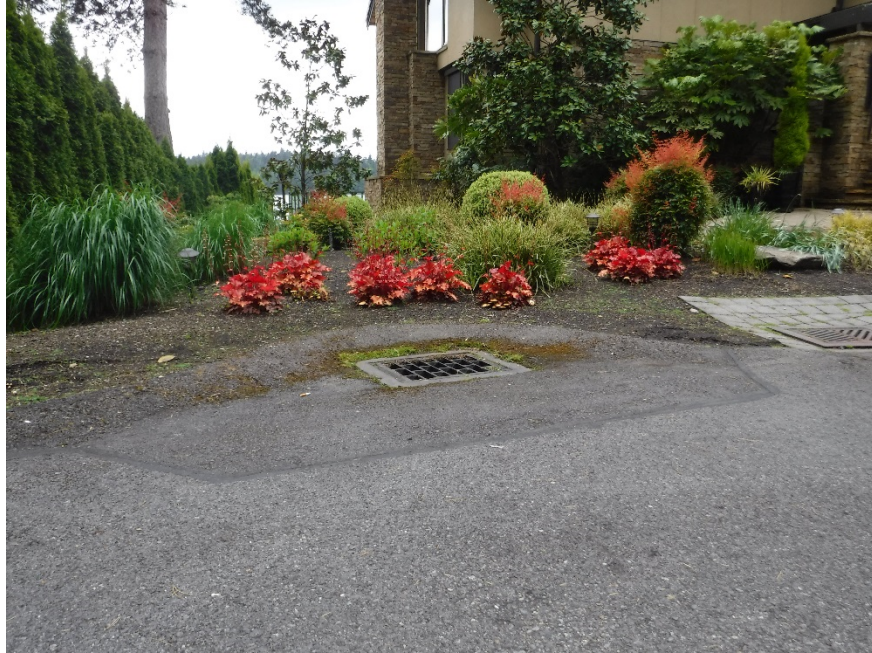
Image 9: 24" concrete culvert pipe enters this CB and flows continue in the westerly direction via 30" corrugated aluminum pipe through a private drainage easement located at 5067 SE 51 st St
