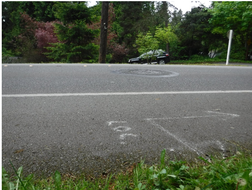
Image 2: Downstream flows are conveyed northwesterly, crossing W Mercer Way via 12" concrete culvert
