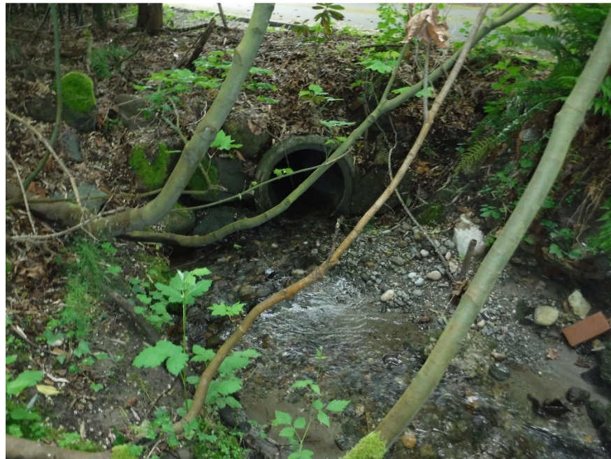
Image 8: Open channel flows inlet this 24" concrete culvert
